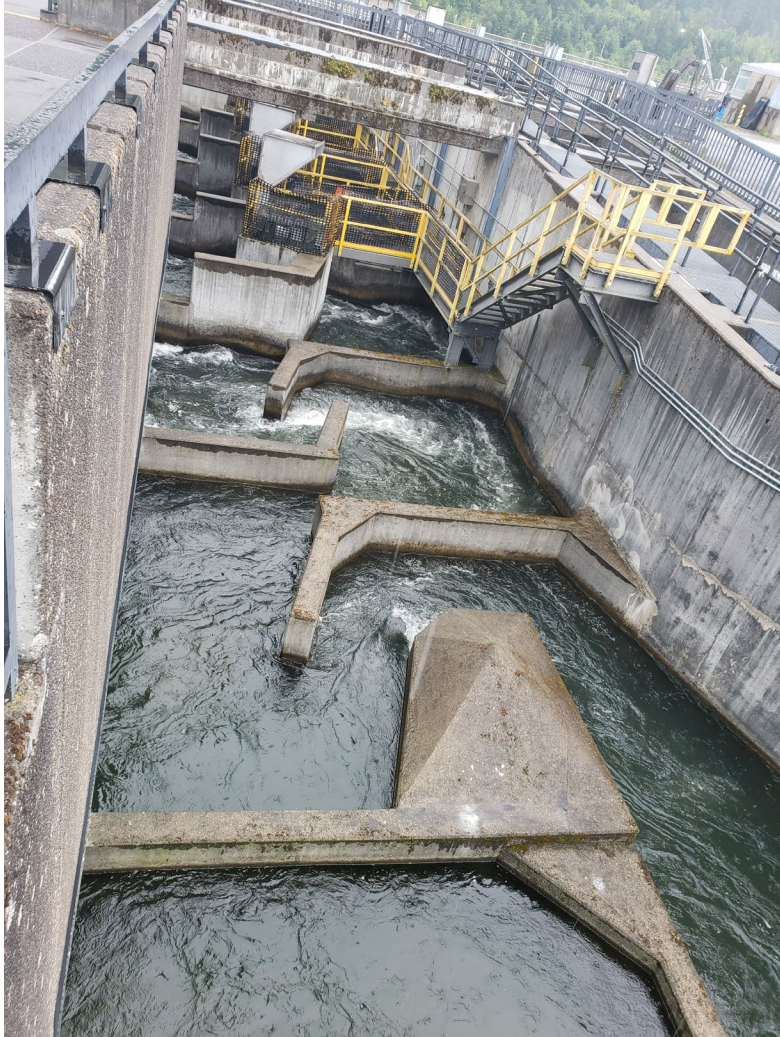
Vertical slot & orifice configuration
