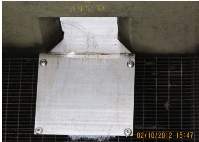
Plating over diffuser grating for attachment
