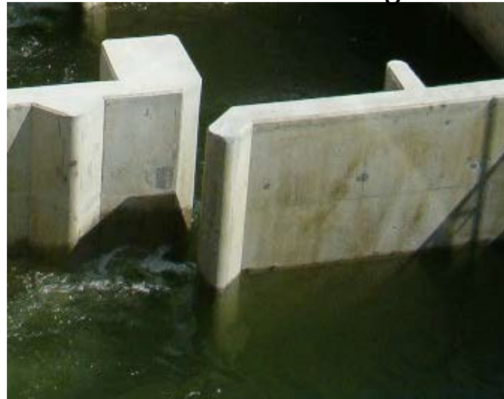
Vertical slot & orifice configuration
